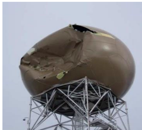
Figure 2. Reno/Virginia peak dome failure (by NWS Reno Electronics Team).
