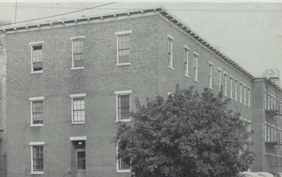
The main brick factory building on Leighton Street, Waterville, is still a glorified ell on the nineteenth century house.
