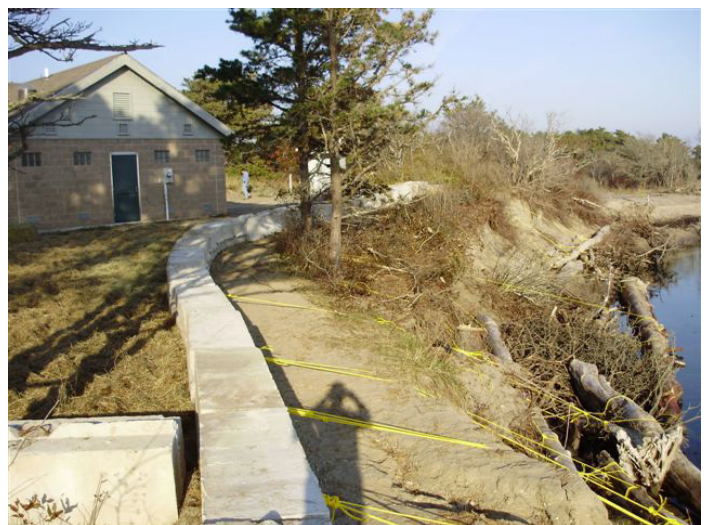
Figure 16b. Placement of jersey barriers for additional splashover protection and to temporarily help anchor rafted trees. Images by S. Dickson, MGS.
