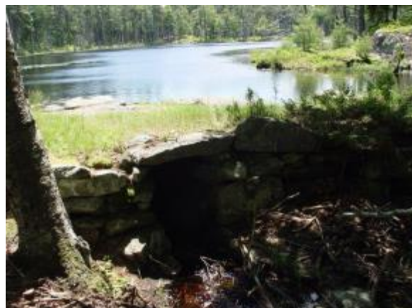
Ice Pond with quarry stone dam in foreground
