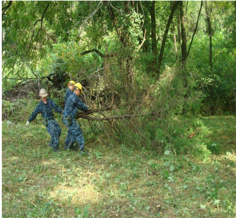
Figure 2.4. United States Navy Seabees Clearing the Site
