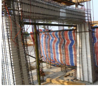
(a) Reinforcement cage of a bridge tower
