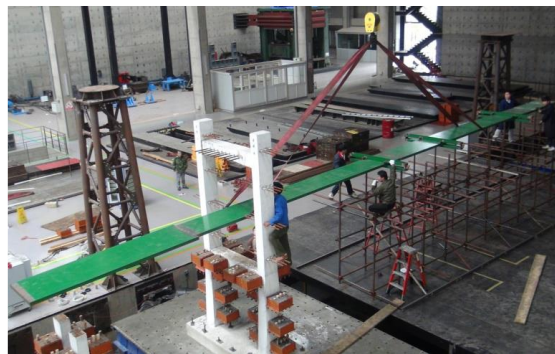
(g) Placement of the bridge girder
