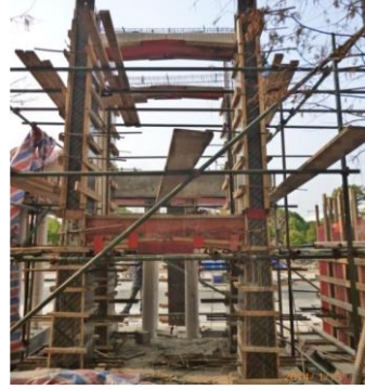
(b) Establishment of concrete formwork
