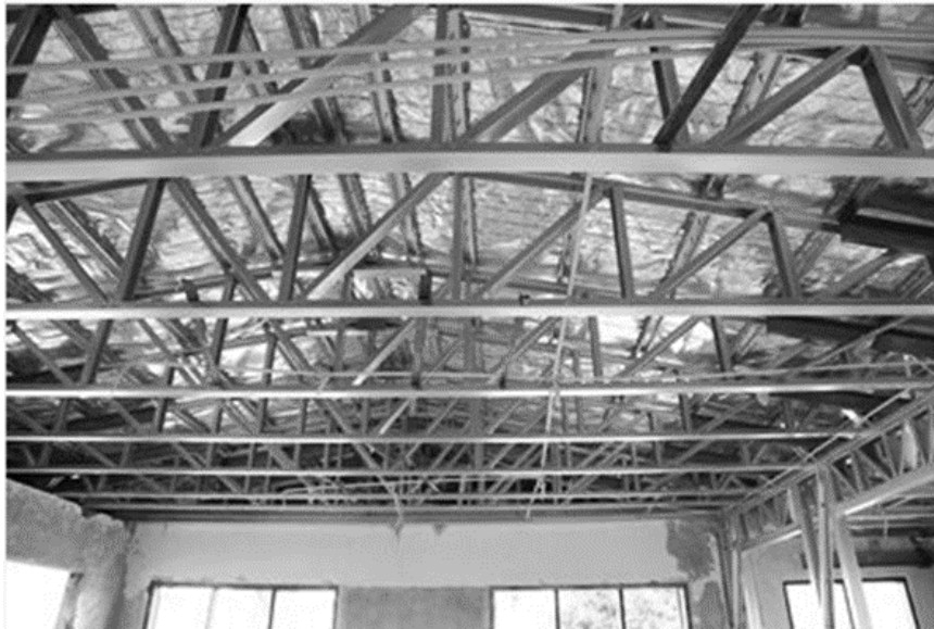
Figure 1 Typical Cold-Formed Steel Roof Trusses (courtesy of FRAMECAD)
