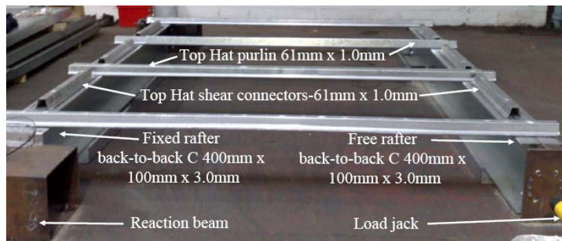
a) Front view – bare roof panel
