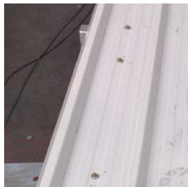
c) Cladding/shear connector
