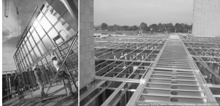
Figure 1: Cold-Formed Steel Framing
