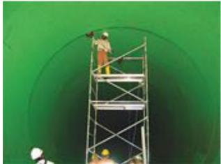
Measure thickness of concrete layers
