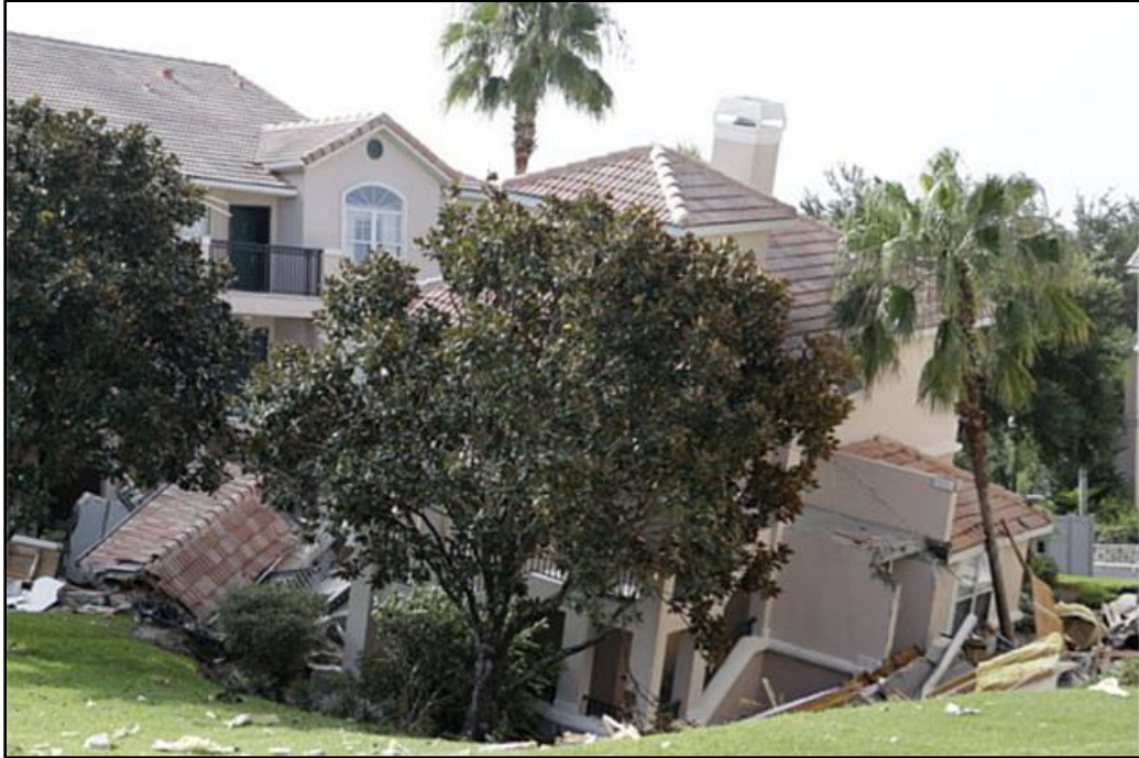
Figure 2.7. Buildings collapse into a sinkhole at Disney World in, Florida. ( http://www.csmonitor.com/Science/2013/0813/Sinkhole-Disney-World-visitors-walking-on-hole-ground ).
