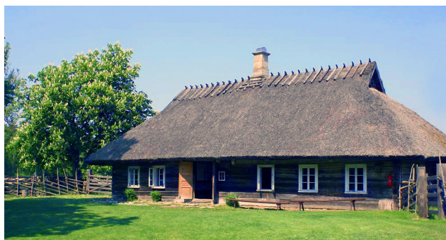
Fig. 11. The main dwelling-house, photo T. Raukas
