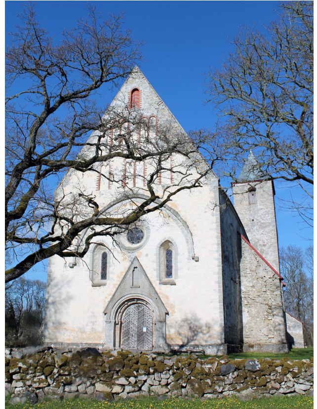
Fig. 9. Valjala Church with visible stone wall made of granite erratic boulders, photo J. Lach
