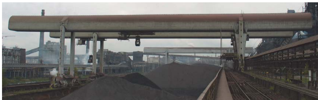
Fig. 1. Gantry cranes of a coating structure
