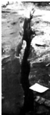
Fig. 3. Vertical fracture plane generated from presplit blasting, adapted from study by Konya and Walter [7].
