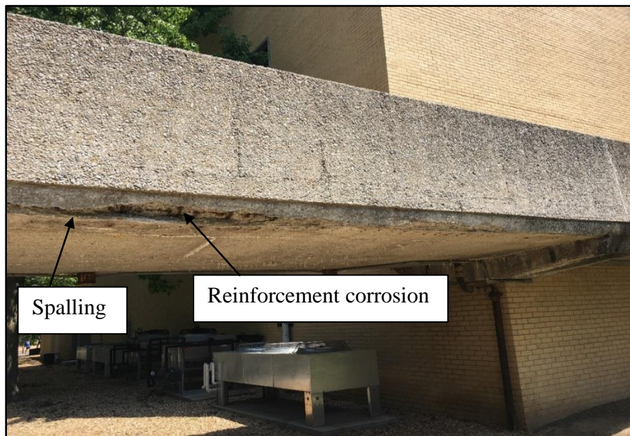
Figure 5.2. Spalling and reinforcement corrosion at the bottom surface of the bridge deck.
