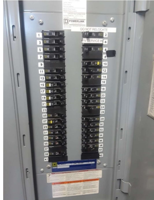
Figure 3.13. Chameleon home circuit panel
