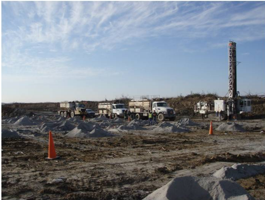
Figure 2.5. Grid of blastholes filled with ANFO. Note gray mounds denote excess nitrogenous chemical around each blasthole.
