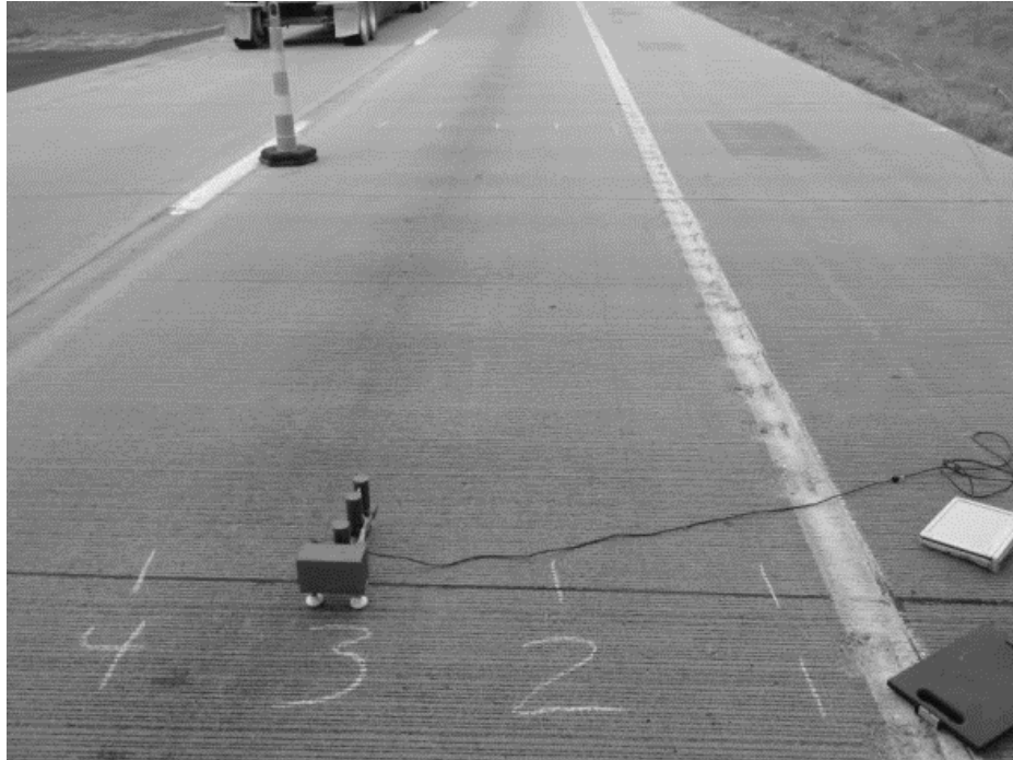
Figure 4. Photo of experimental site.
