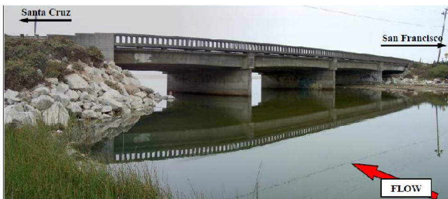
Figure 2.5. Highway 1 Waddell Creek Bridge.
