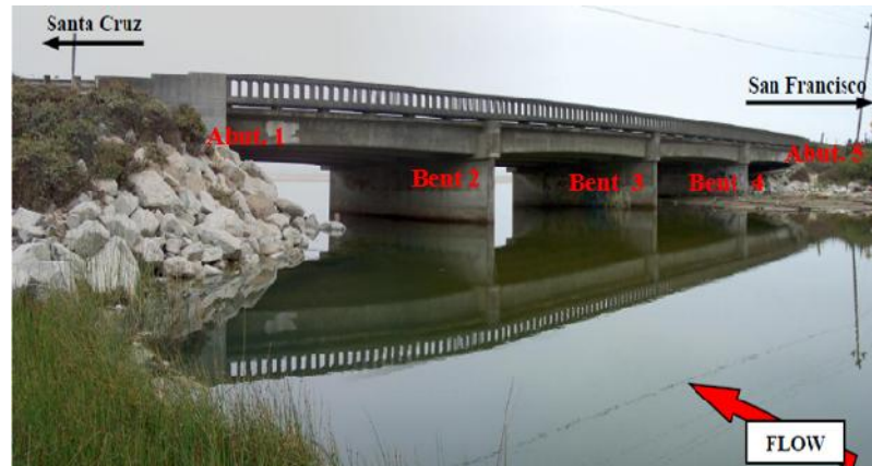
Figure 5.12. State Highway 1 Bridge over Waddell Creek, CA.
