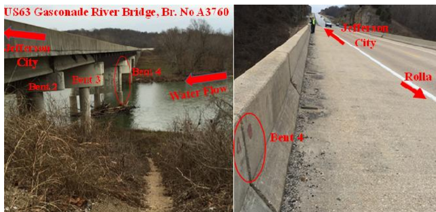
Figure 5.22. The US Highway 63 Gasconade River Bridge.
