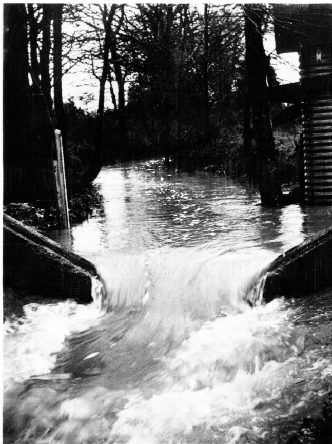
FIG. 4 RIGHT STAFF GAGE AND RECORDER INSTALLATION
