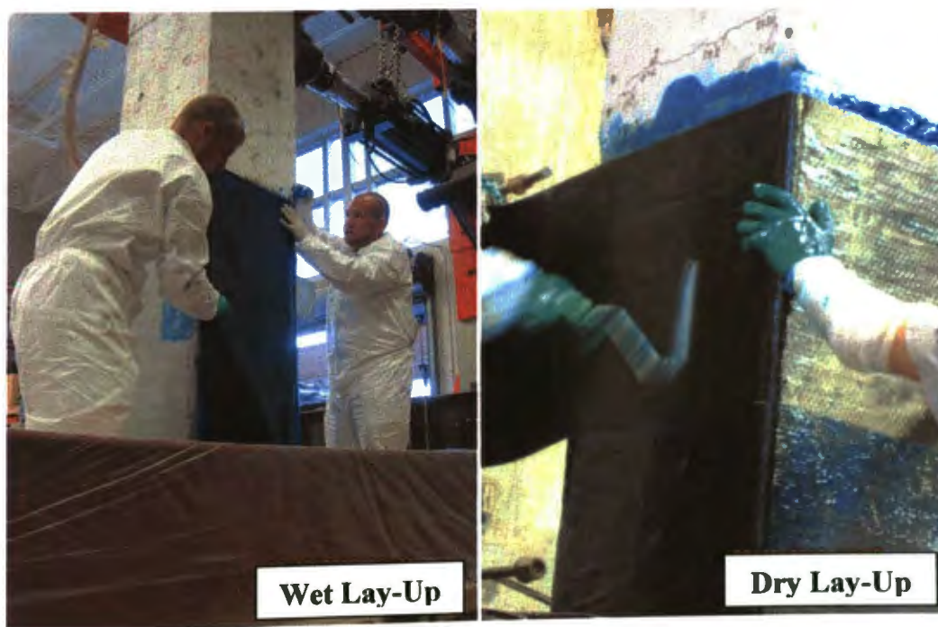
Figure 4.21. Installation of CF 130 Carbon Fiber Sheets
