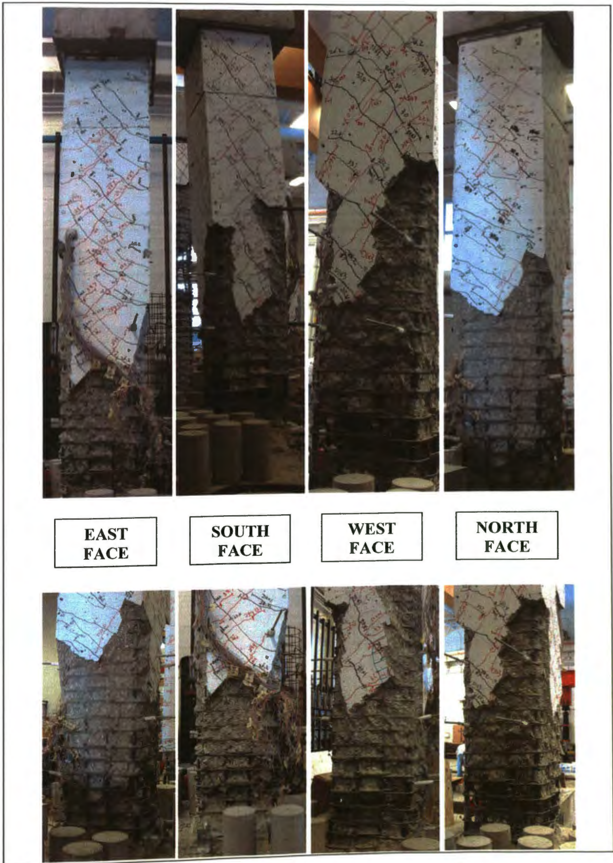
Figure A-3. Damage Photos of Column #3 Prior to Repair
