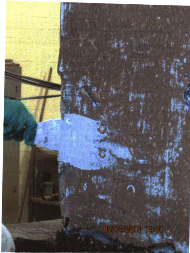
Figure 4.20. Application of MBrace ® Putty
