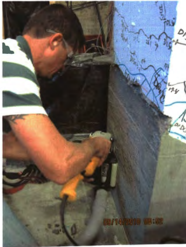
Figure 4.18. Concrete Surface Preparation
