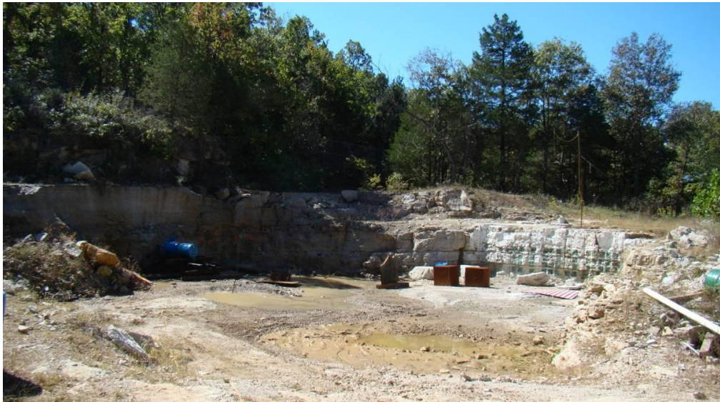
Figure 4.1 Above Ground Testing Facility
