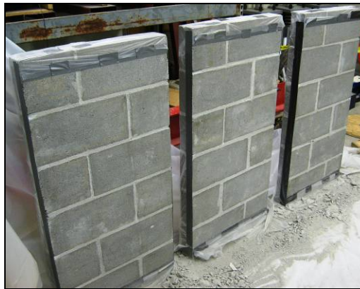
Figure 6.2. Phase 2 URM Walls Prior to Strengthening
