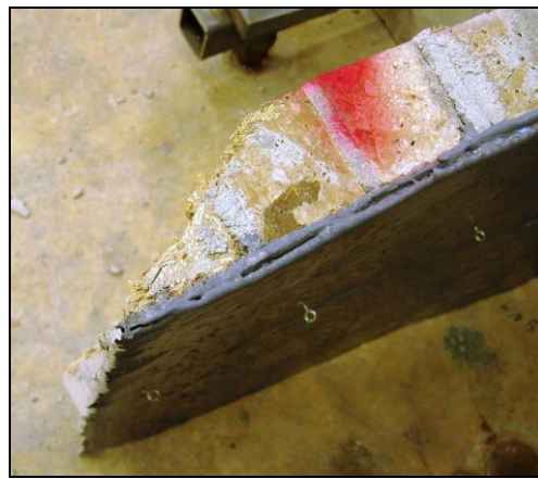
(b) Damage Sustained to WF-FA Units
