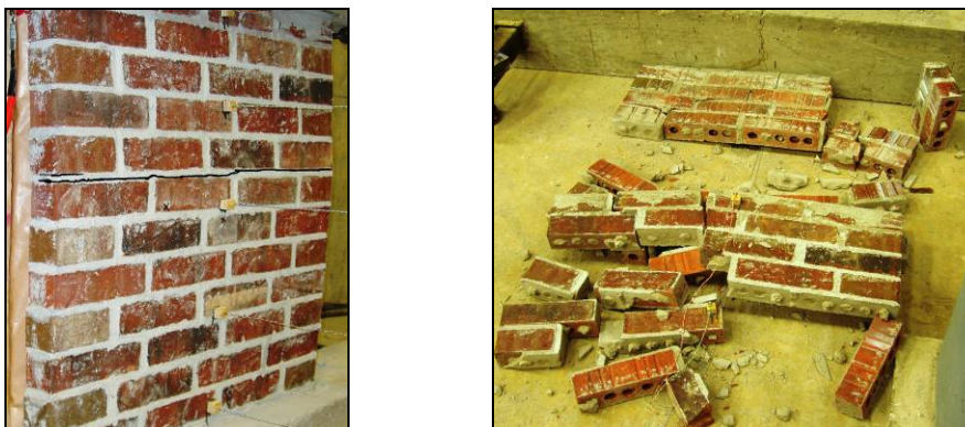
(a) Horizontal Crack
