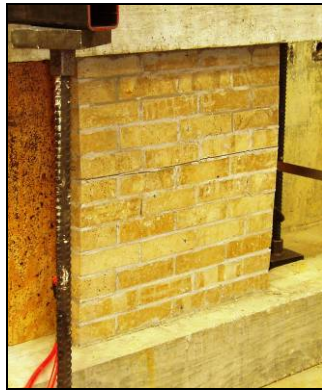
(a) Horizontal Cracking
