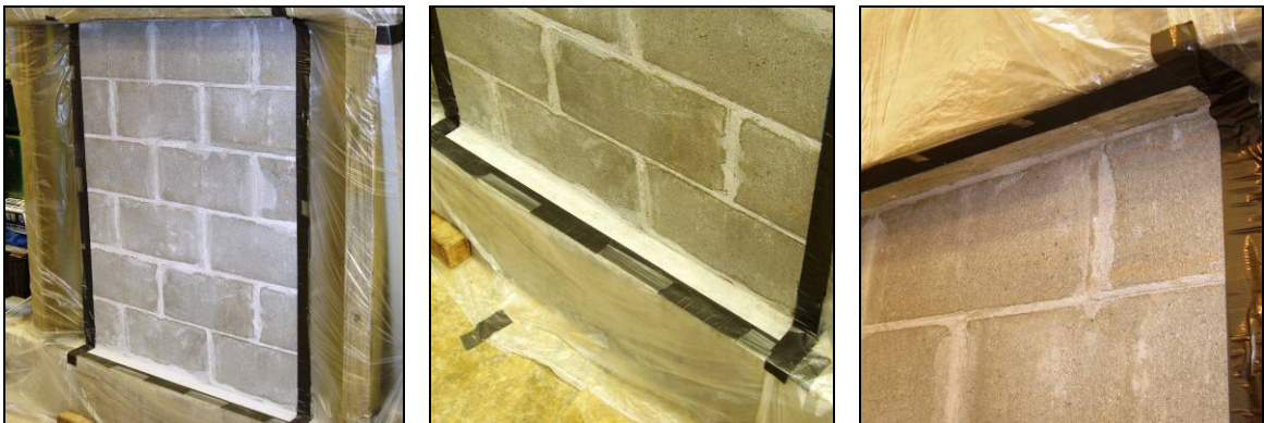
(a) Face of URM Wall
