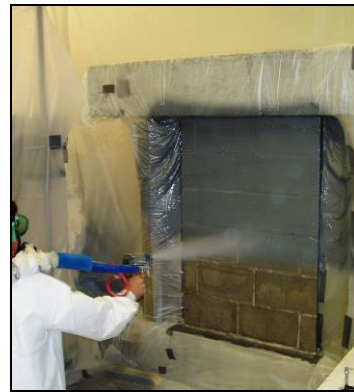
(b) Application of Polyurea
