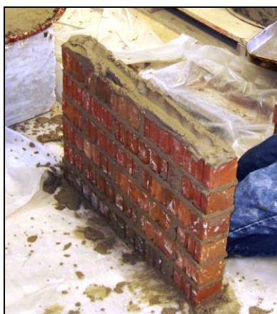
(c) Bed-Joint Construction
