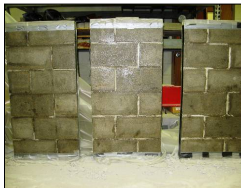
(b) Primed URM Walls
