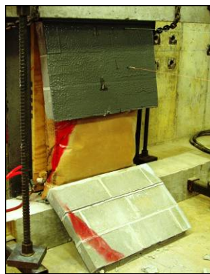
(c) Wall Failure
