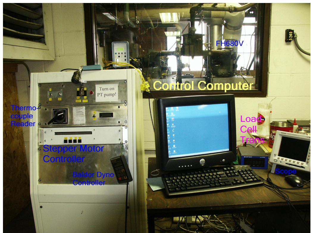
Figure A.3: Control room for vertical dyno.
