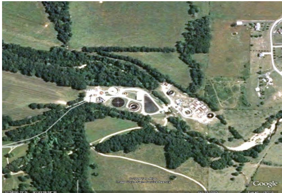
Figure 5.1. Aerial View of Rolla Southeast WWTP
