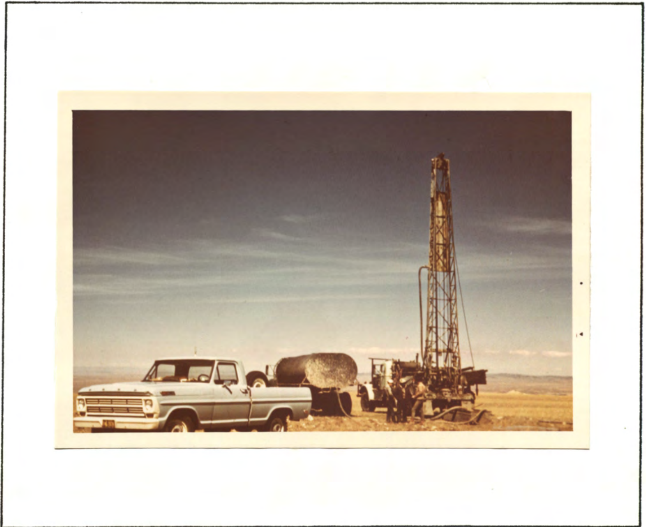
Frontispiece. Drilling rig in operation, Poison Spider Area, Wyoming.
