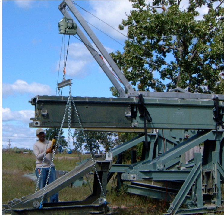
Figure 4.19: First Crane System Design Performing a Bottom Panel Lift
