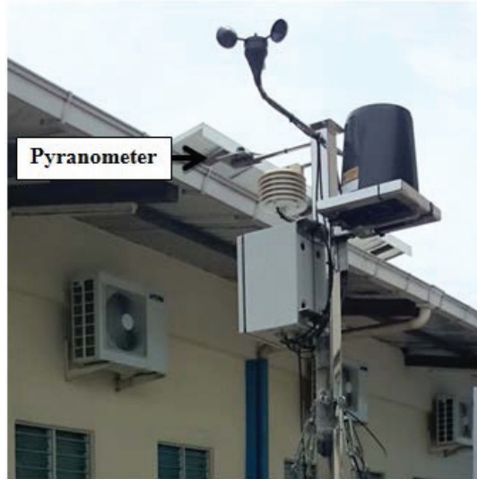
Figure 1. Weather station at Kompleks Makmal FKM UTeM
