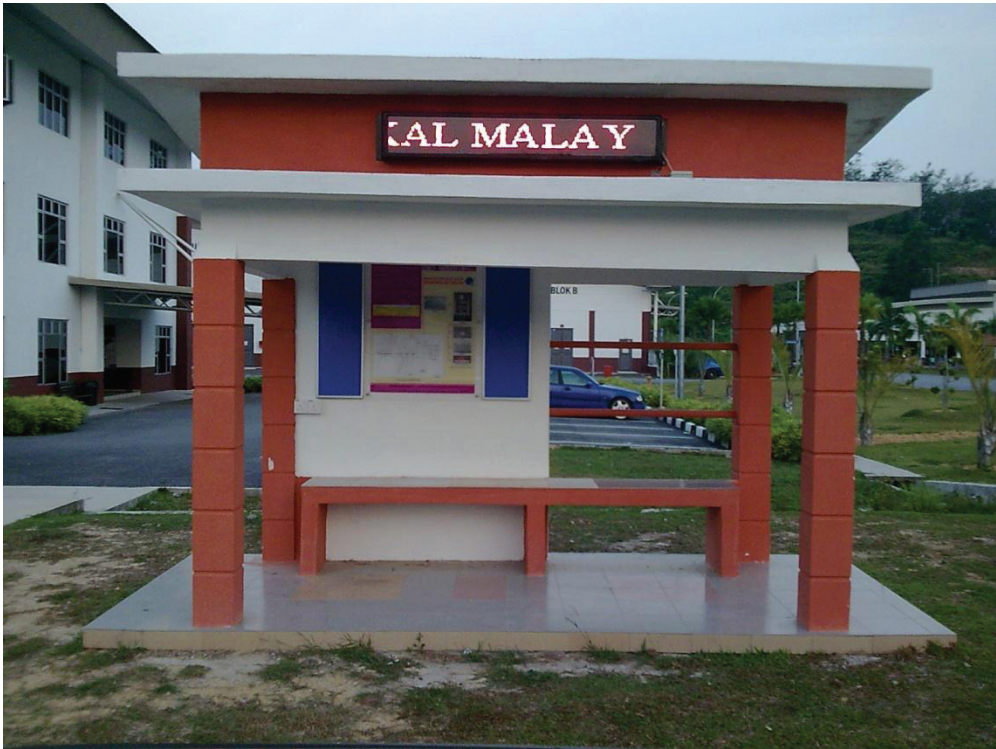
FIGURE 6 UTeM Stop with Stand-alone PV System
