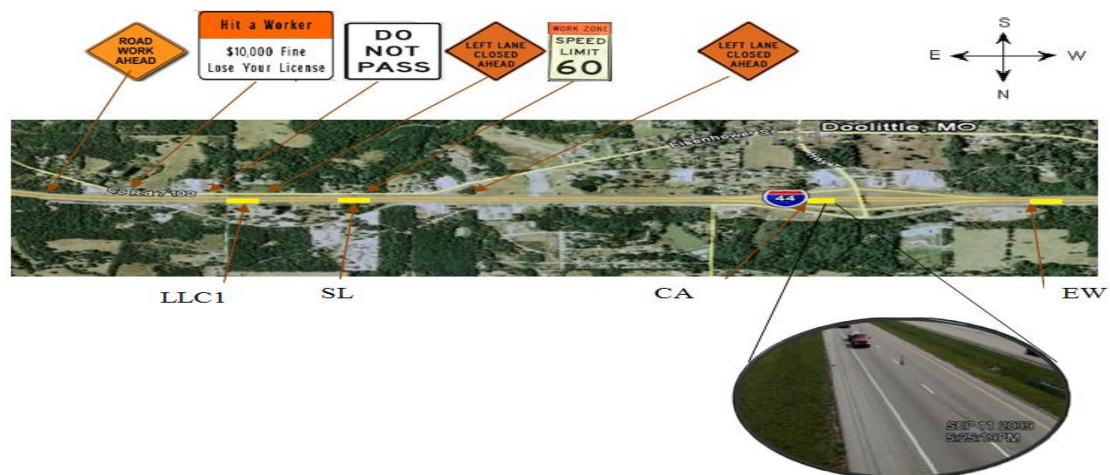
(c) Aerial View of I-44 WB and Location of Signs, Camera View of Data Collection Site
