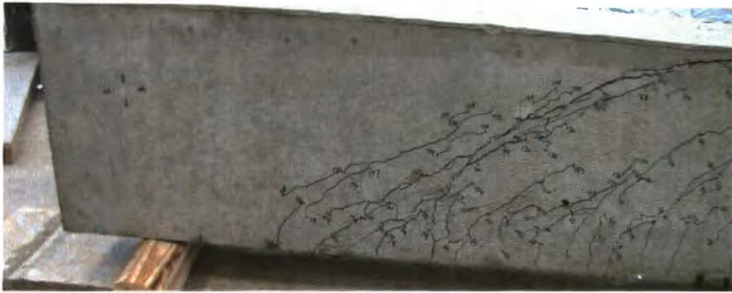
Figure 6.55. SCC-7-1 Beam at Failure
