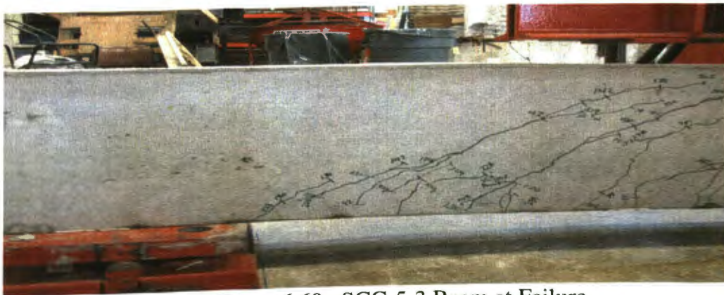
Figure 6.60. SCC-5-3 Beam at Failure
