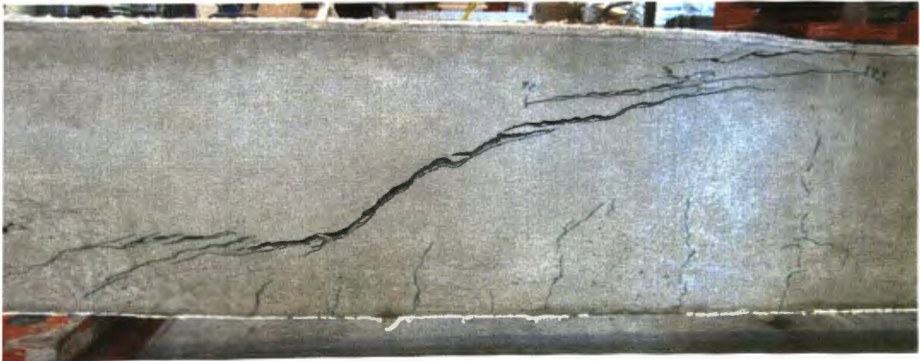
Figure 6.53. SCC-NS-2 Beam at Failure
