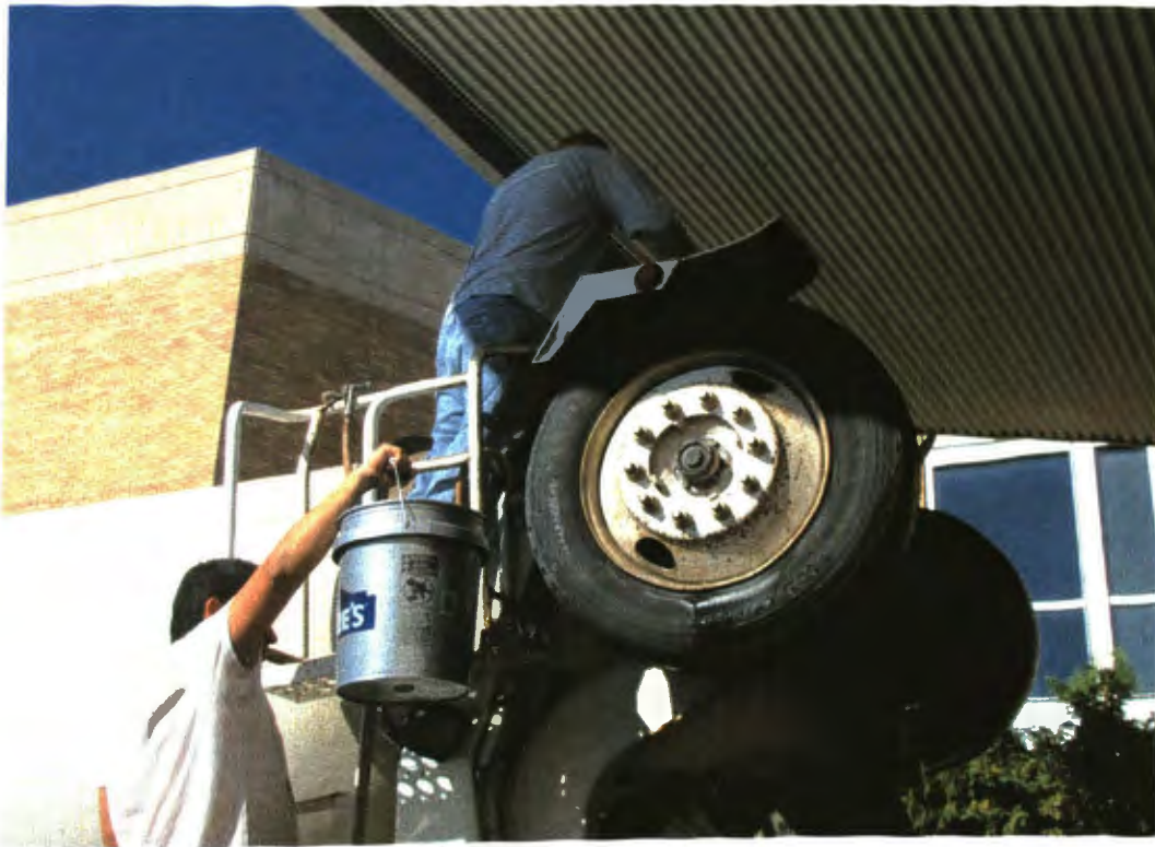
Figure 6.14. Addition of Chemical Admixtures
