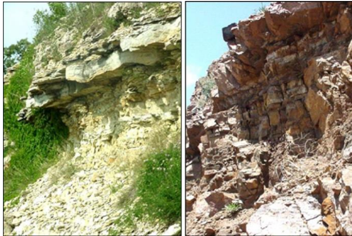
Figure 2.5. Two types of raveling that are caused by weathering of rocks and removal of soft material (Maerz, 2012)
