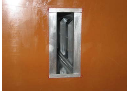
Figure 3.33: Silicone added to fill any voids
