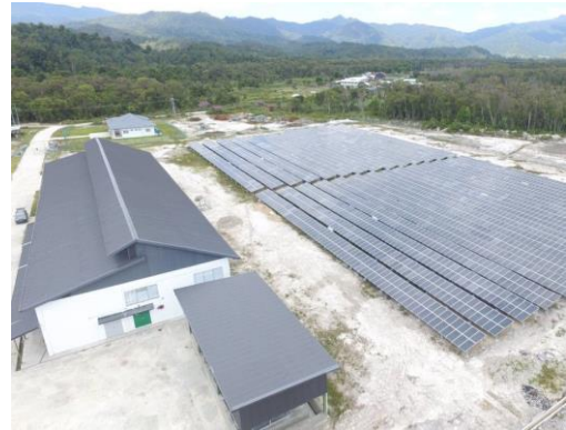
Figure 2: Centralized Solar Hybrid System in Bario [10].
