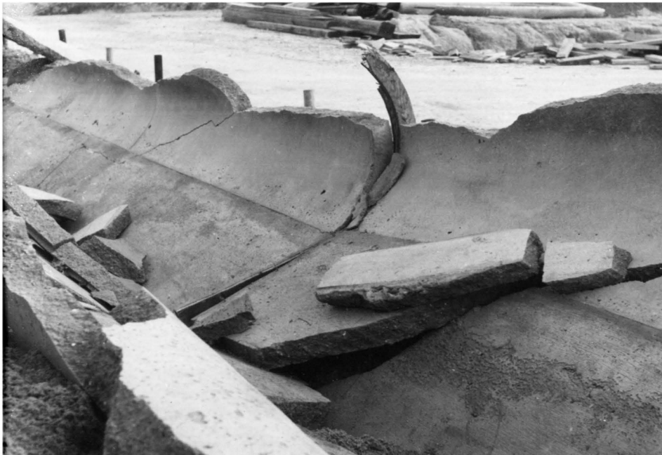
Figure 57. The Phase IV tunnel after demolition.
