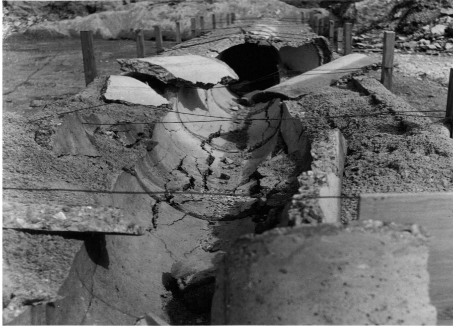
Figure 62. The results of demolition, Test Two, Phase VII.
