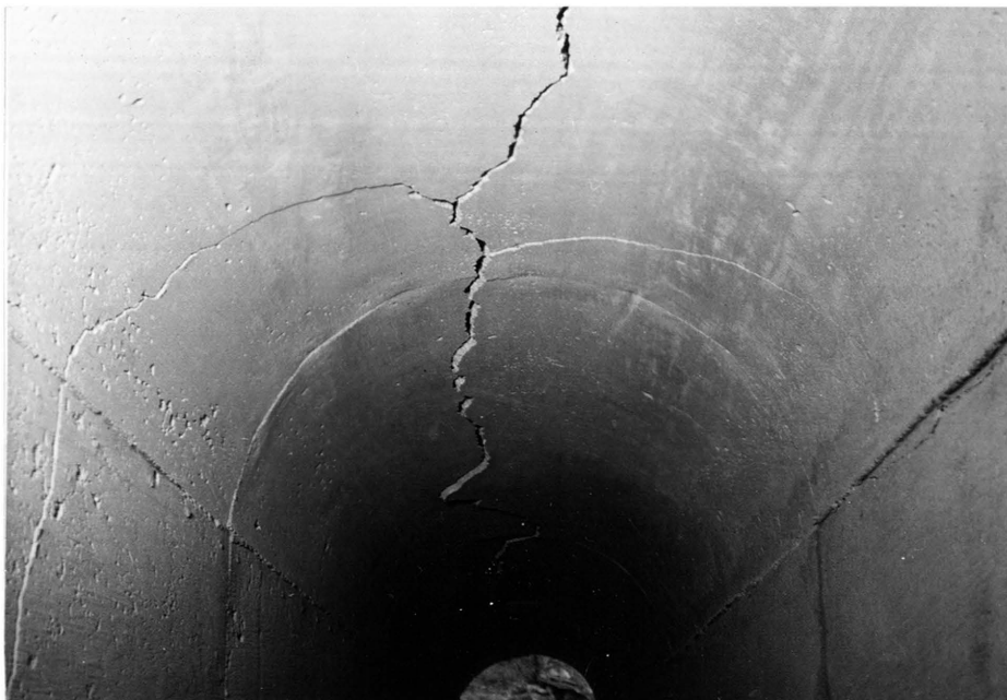
Figure 39. The results of demolition in Test Six "A", Phase II. The picture taken from the east portal.
