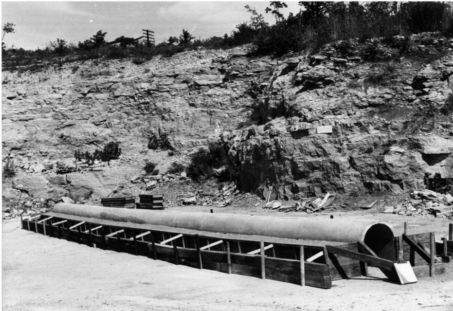
Figure 33. Type A tunnel constructed for Test Five, Phase II.
