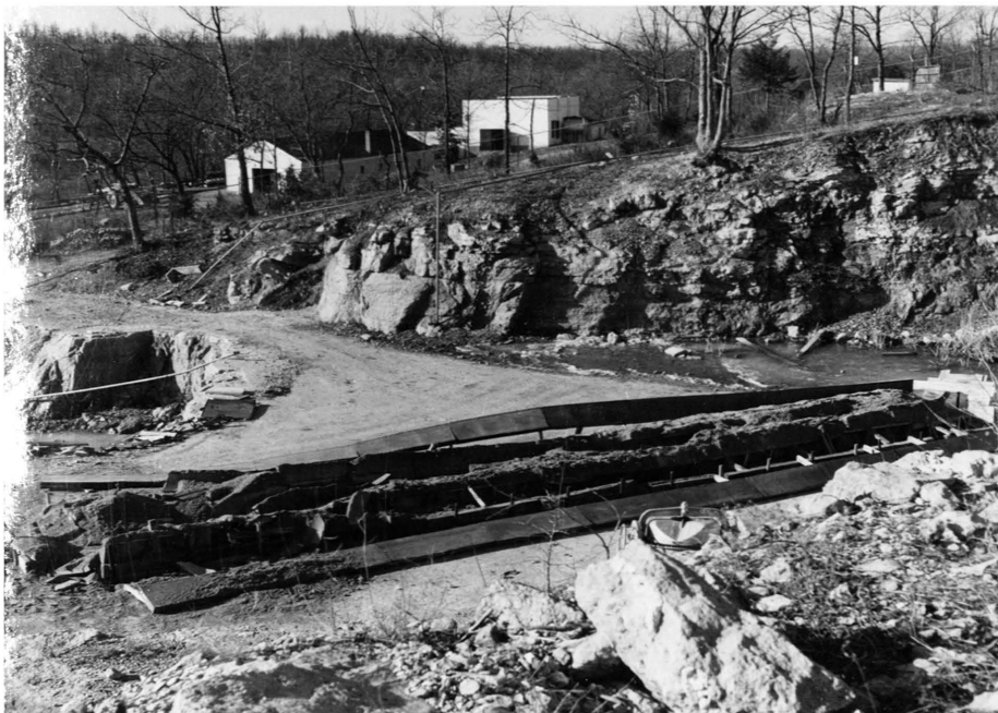
Figure 55. The results of demolition in Test Six, Phase III.
