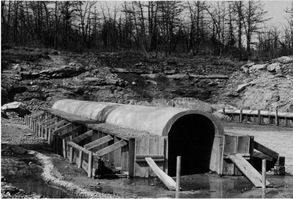
Figure 58. The Type B tunnel constructed for Test Two, Phase V.
