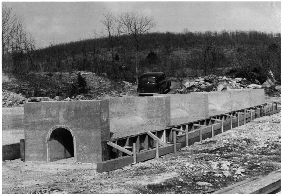
Figure 45. The tunnel which was constructed for Test Eight, Phase II.
