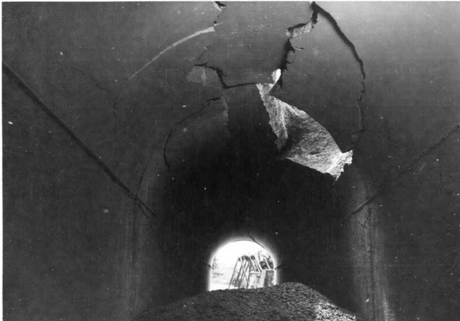
Figure 40. The results of secondary demolition in Test Six "B".
