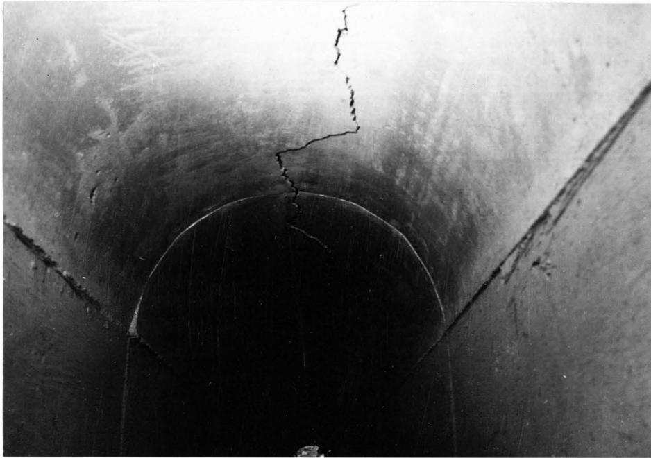
Figure 42. The results of demolition in Test Seven "A", Phase II. The picture was taken from the east portal.
