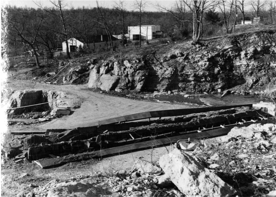
Figure 54. The results of demolition in Test Six, Phase III.
