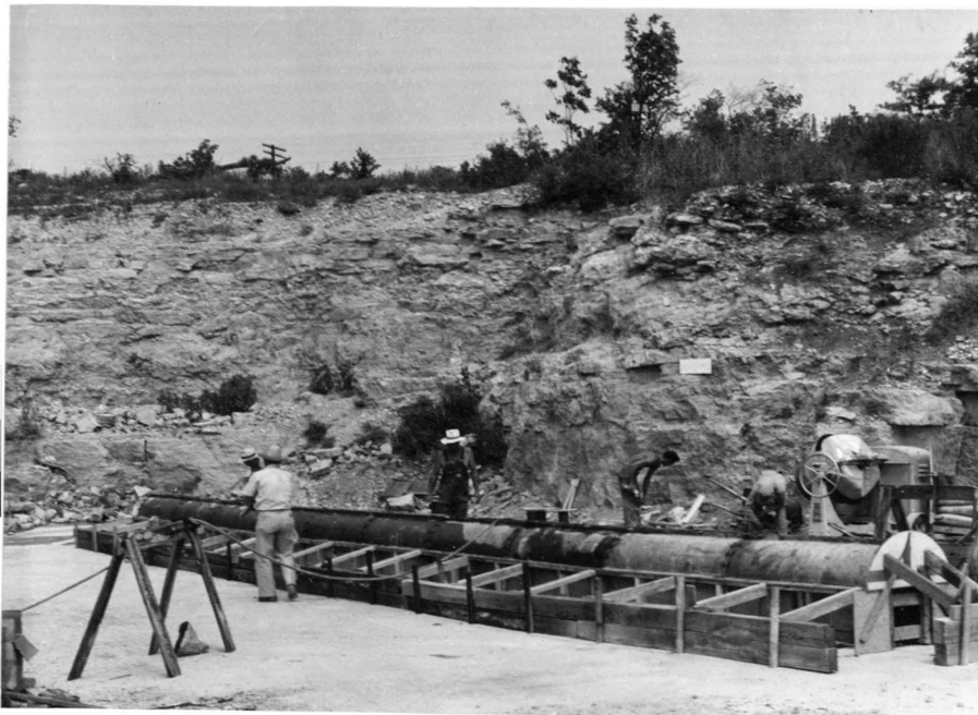
Figure 6. Outside metal arch forms joined together with machine bolts.
