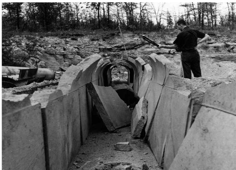
Figure 60. The results of demolition in Phase VI.
