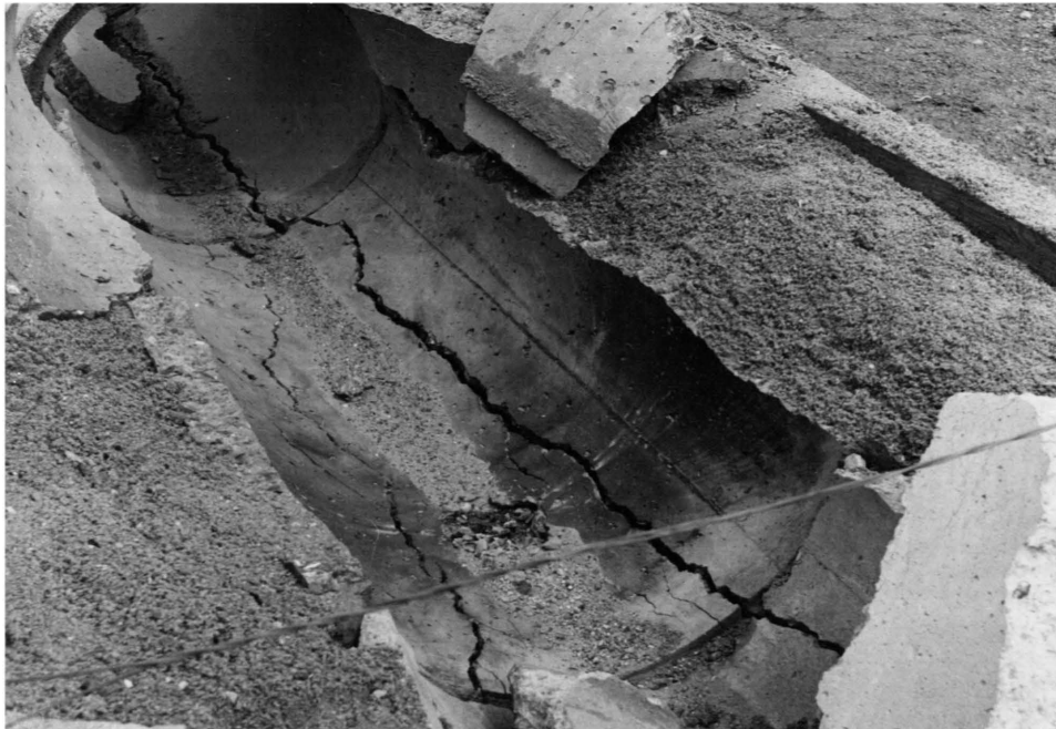
Figure 67. The results of demolition in Test Two, Phase IX.
