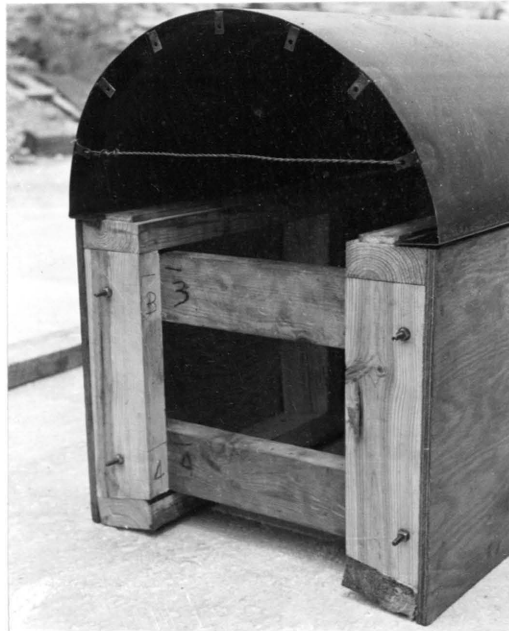
Figure 4. Inside metal arch forms.
