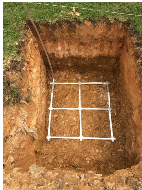
Figure 3: Microgrid installation without additive.
