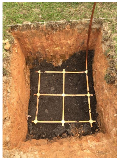
Figure 4: Microgrid installation with additive.
