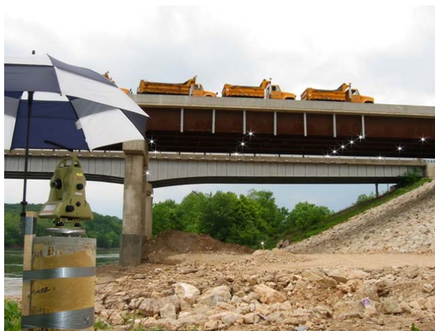
Figure 7 – ATS setup: (a) schematic of location of targets; (b) reflecting prism; and (c) photograph of setup with total station. Dimensions in m.
