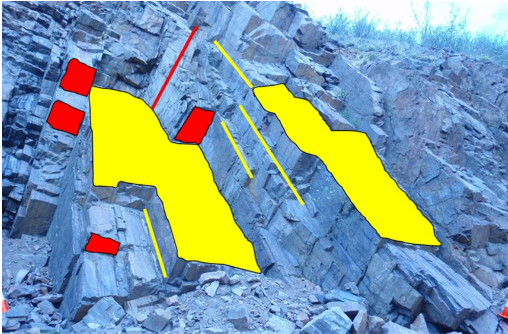
Figure A.17. Non-vertical rock face showing a trace (red line) and facets (red rectangles) belonging to the same set.
