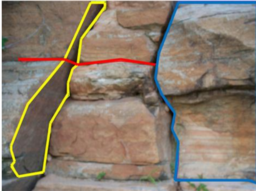
Figure 4.1. Image of a rock cut showing a natural facet (yellow polygon), a trace (red line) and a blasted facet (blue polygon).
