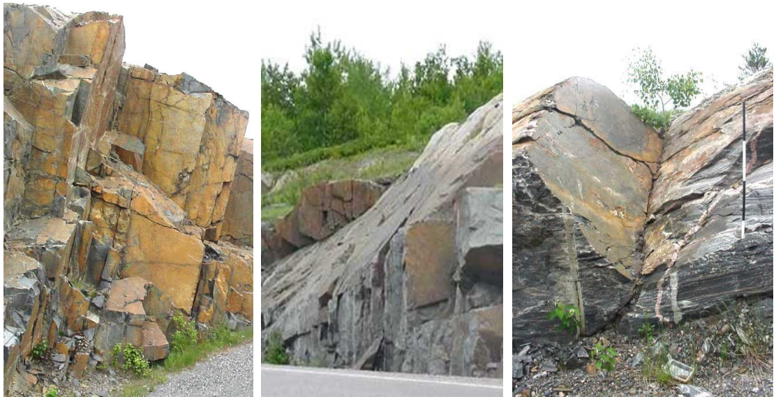
Figure 2.5: Example of toppling, planar, and wedge rock failures respectively along highway rock cuts (Retrieved from Maerz & Kim, 2000).
