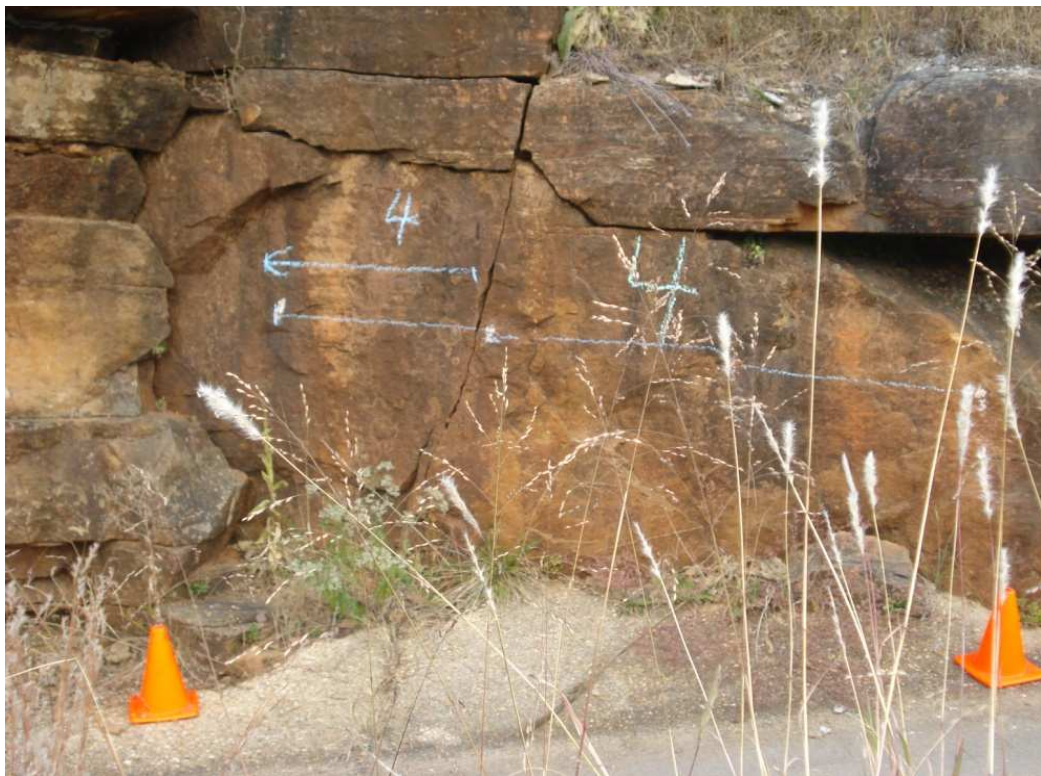
Figure 6.13: A front view of the rock slope of St.4 in site 1.
