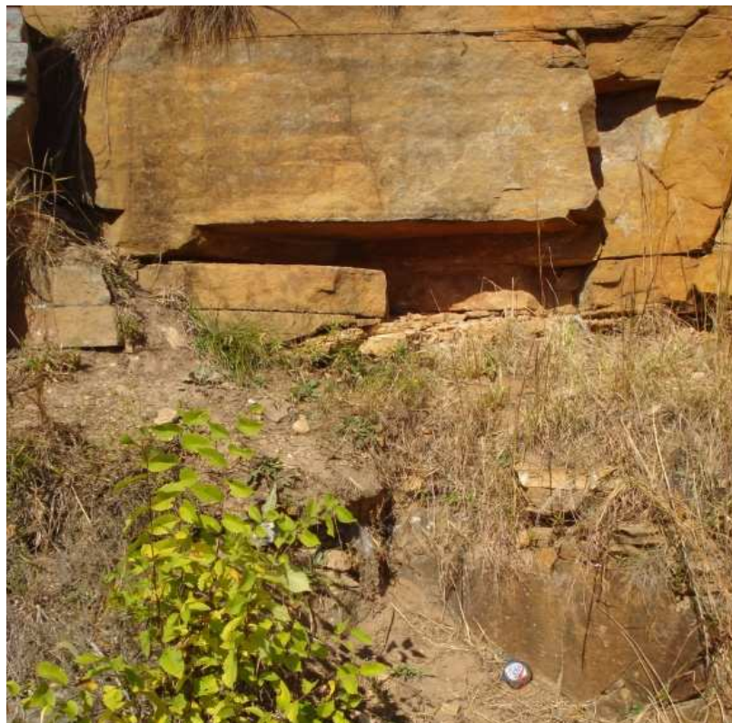
Figure 6.17: A front view of the rock slope of St.5 in site 1.
