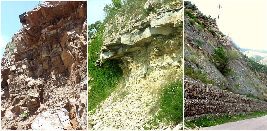
Figure 2.4: Raveling, undercutting, and rolling failures along Highway 70 road cuts, respectively, Colorado State, USA (Retrieved from Maerz & Kim, 2000).
