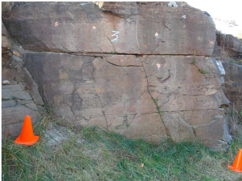
Figure 6.9.: A front view of the rock slope of St.3 in site 1.
