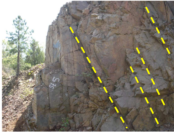
Figure 2.8: A potential toppling failure at station 7 in site 2 of the study area. Notice that the potential sliding planes of some discontinuities (dashed yellow lines) are dipping steeply into the rock slope.
