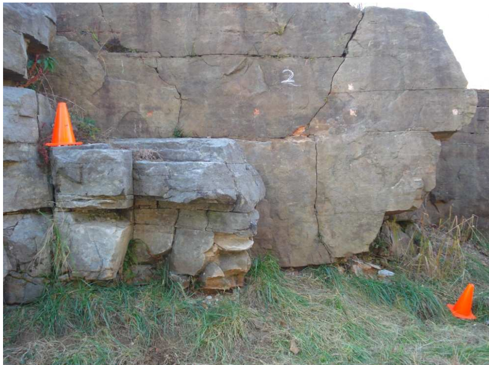
Figure 6.5: A front view of the rock slope of St.2 in site 1.
