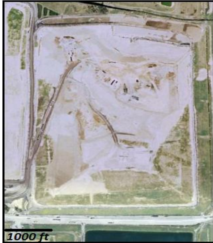
Figure 3 – Aerial image of the Seneca Meadows landfill.
