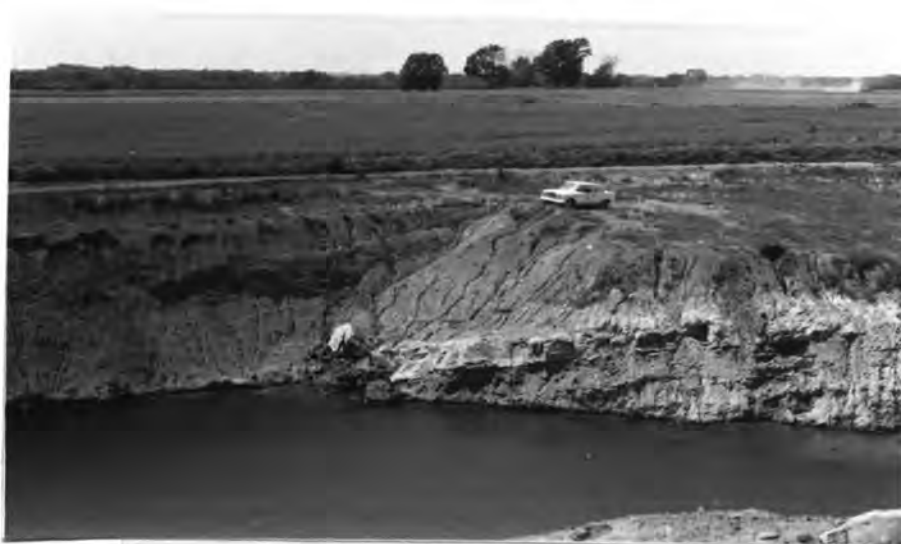
Figure 21. Disturbed strata in west highwall of abandoned coal strip mine at Stratigraphic Section No. 15, north-central Vernon County. Light-gray bed near center of photo is 4 ft. thick and is composed of sandstone. It underlies the Croweburg coal in the Rich Hill area. The Mineral coal was mined. Structurally the section is on the southwest flank of the Schell City-Rich Hill anticline. Dip is 30^{\circ} S, 45^{\circ} W. Photo taken looking west.
