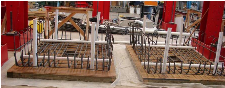
Figure 3.14 Assembly of Bottom Mat of Reinforcement for Foundation
