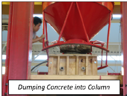
Figure 3.18 Concrete Pour for Foundation and Column
