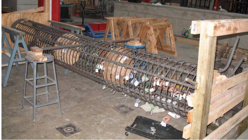
Figure 3.13 Fabrication of Column Cage
