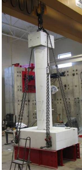
Figure 3.19 Fabricated Column at Temporary Location for Inserting Axial Tendons
