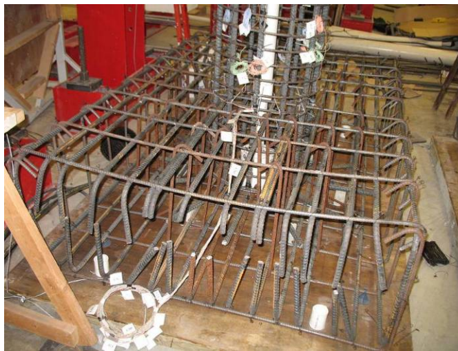
Figure 3.15 Finished Foundation Reinforcement with Column Cage
