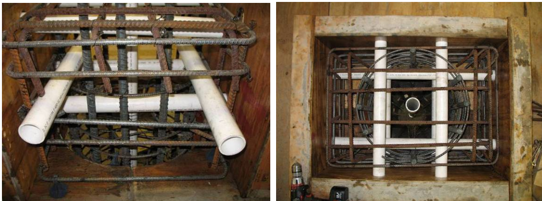
Figure 3.16 Formwork and PVC Layout on Loading Block
