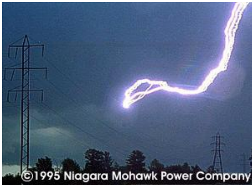
Figure 2: Lightning flash to an overhead power line of a high voltage power transmission grid [3]
