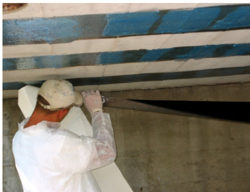
(c) Application of CFRP laminates
