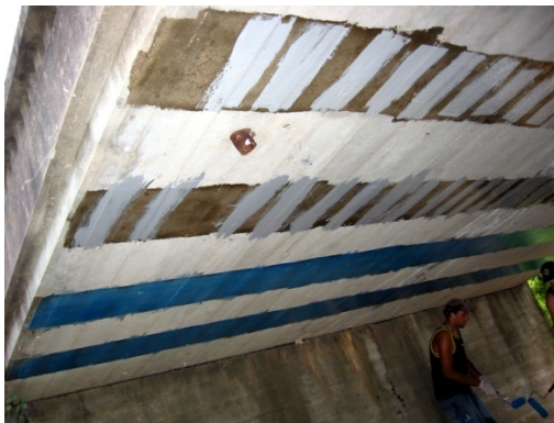
(a) Surface preparation with primer and putty
