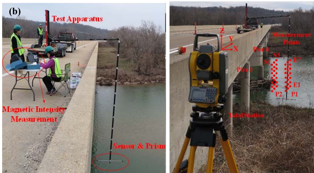
Figure 5.22. US63 Bridge site: (a) planning (unit: m), and (b) test setup.
