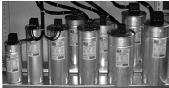
Fig. 3. Capacitor models (with various capacities) which set the 'heart' of each battery used for reactive power compensation
