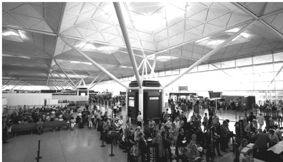
Fig. 1. London-Stansted Airport terminal, designed by Norman Foster. Terminal is roofed by a lightweight canopy structure, allowing natural insulation, daylight penetration and natural ventilation of the building. Source: http://www.si.wsj.net/
