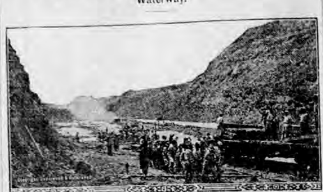
How the Floor of Culebra Cut Was Cleaned in Readiness for the Flooding of the Panama Canal.
