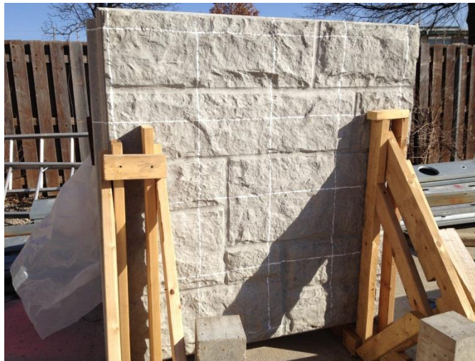
Figure 2.1 Erected MSE wall used in this investigation
