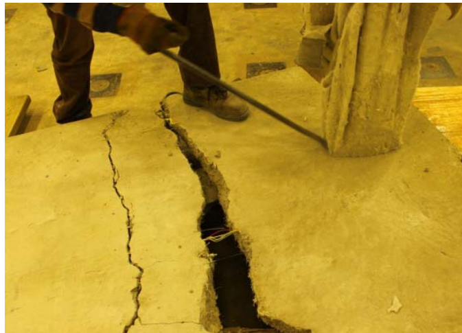
Fig. 6.3. Removal of the fabrics from concrete panel.
