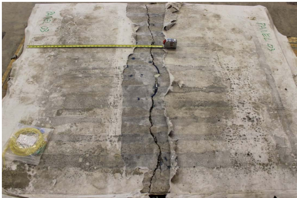
Fig. 6.8. Cracks in P3 after load frame test.
